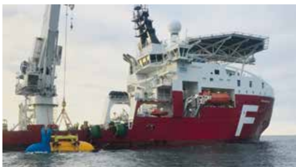
Re-installation of the Sabella D10 turbine in the Fromveur Passage
