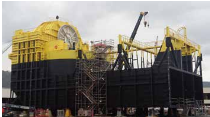
OE Buoy Build December 2018
