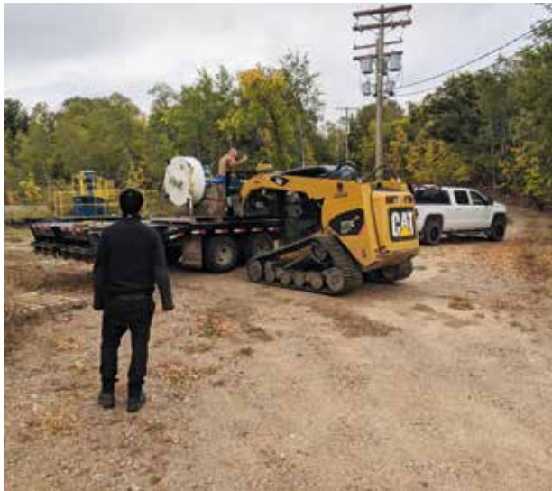
New Energy Corp. Preparing for installation, photo credit: CHTTC
