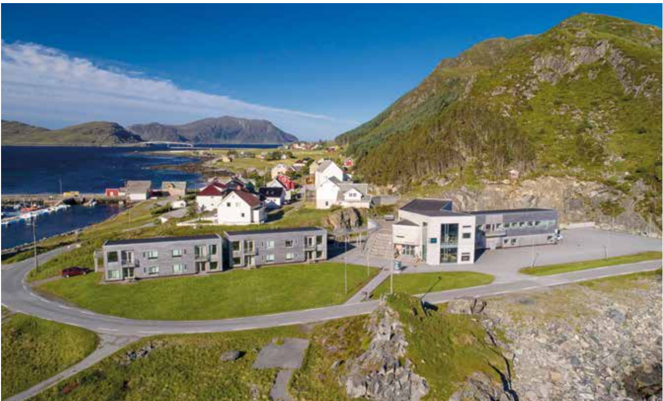
Runde Environmental Centre (REC) at Runde Island on the Norwegian west coast (Photo credit: Per Eide)
