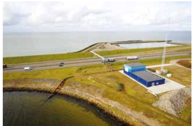
Redstack pilot facility
