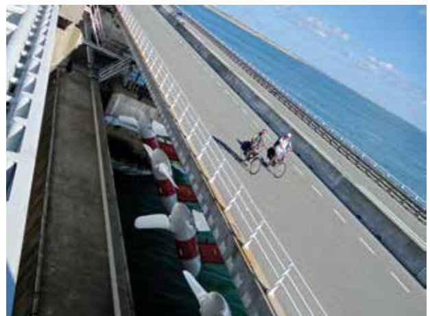
Tocado tidal power plant in the Eastern Scheldt (Photo credit: Tocardo Tidal Power)
