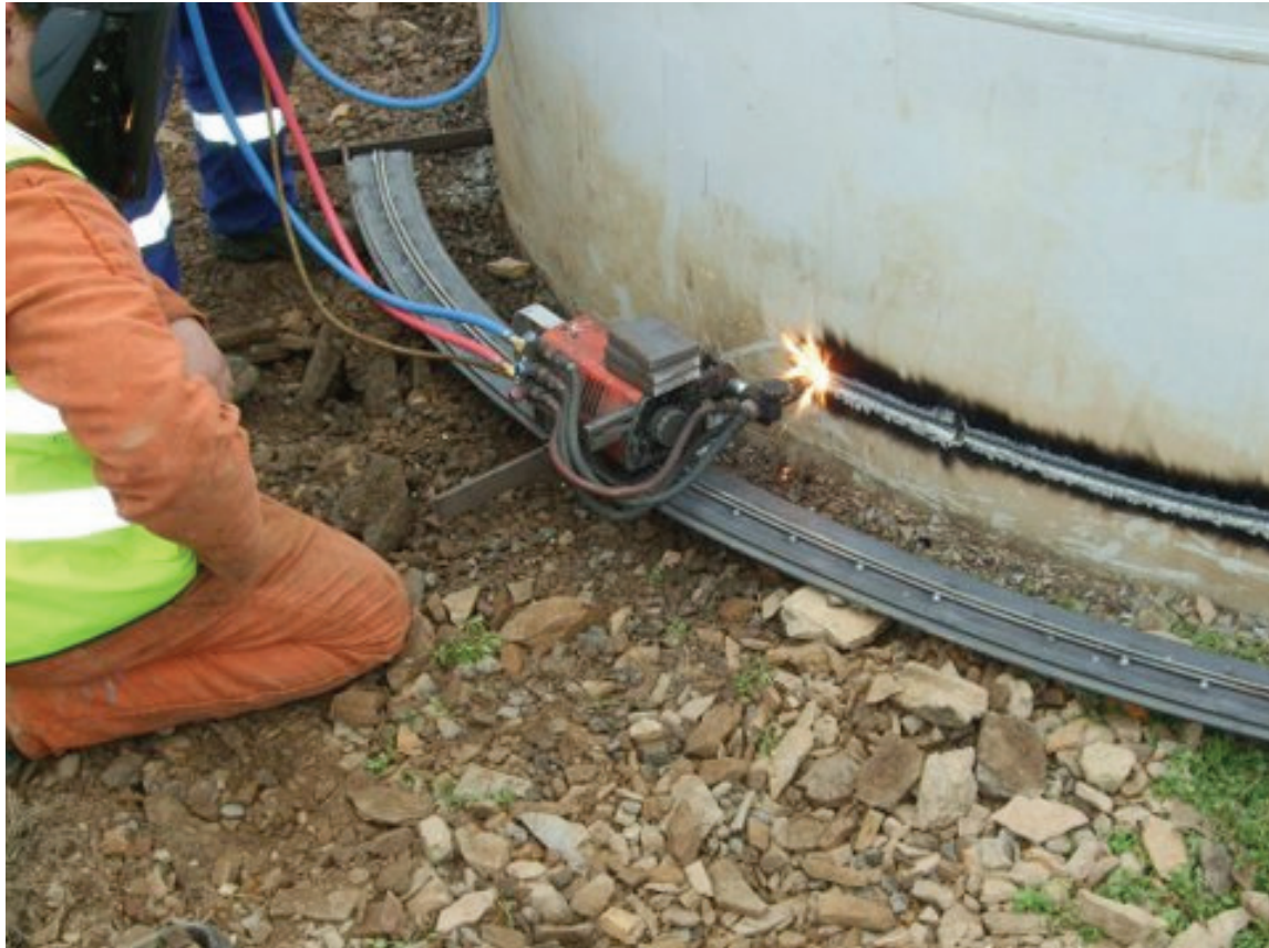
Figure 4: Cutting tower base at Spurness Wind farm, Orkney. Courtesy SSE Renewables.
