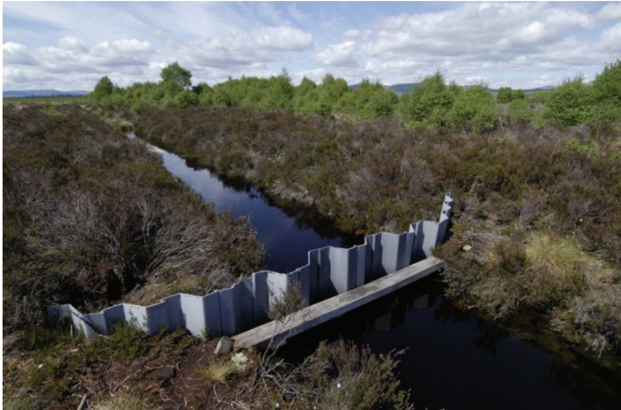
Figure 6: Sheet piling damming a ditch at Flanders Moss ©Lorne Gill/SNH
