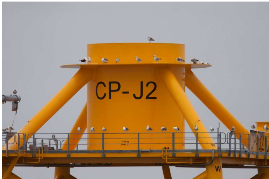
Gulls resting on a jacket foundation at the Thorntonbank during construction of phase II & III (photo: Hilbran Verstraete)
