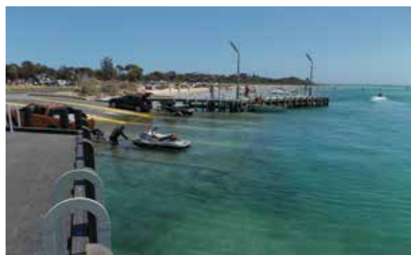
Rye boat ramp, a popular access point to the southeastern area of Port Phillip Bay, was upgraded in 2018 at a cost of $1.23 million. Photo: R Molloy
