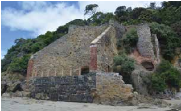
Ruins of lime burners' kilns, Cape Liptrap Coastal Park, Walkerville. Photo: Parks Victoria
