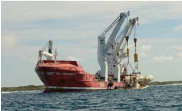
Lifting bioWAVE from installation vessel. Photo: BioPower Systems
