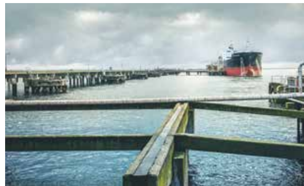
AGL is investigating a floating storage and regasification unit at the Crib Point jetty in Western Port for the importation of liquified natural gas (LNG). Photo: CEE Consulting Environmental Engineers
