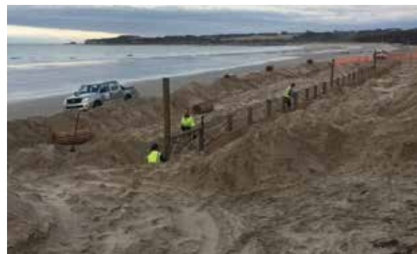
Wet sand fence installed at Inverloch to reduce erosion in front of life saving club. Photo: A Kilborn
