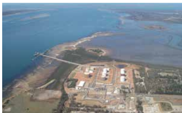
Long Island Point with oil and gas processing plant and wharf. Substantial areas of mangrove and saltmarsh were filled to create land for industrial use. Photo: R Molloy
