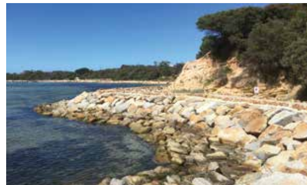
Dorothy Houghton Walk was constructed to reduce cliff erosion at the site of Victoria's first settlement at Sullivan Bay, Sorrento. Photo: Robert Molloy
