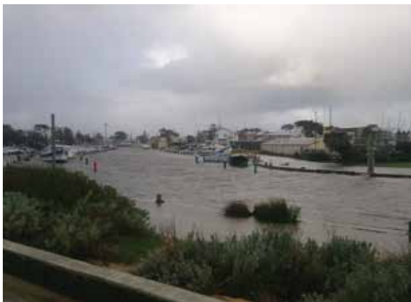
Storm tide at the entrance to Mordialloc Creek, 24 June 2014. Photo: Water Technology
