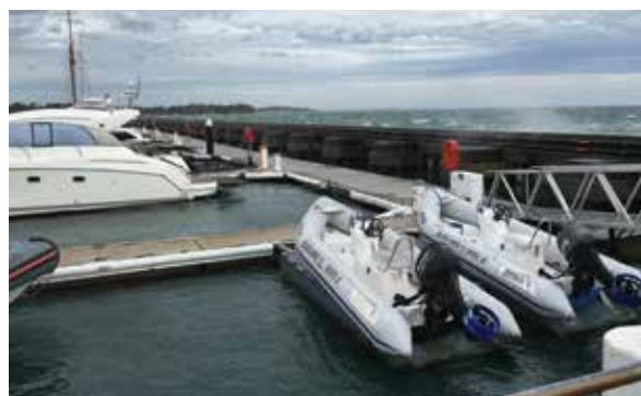
Blairgowrie Yacht Squadron Marina includes components to enhance biodiversity and reduce its ecological impact – these include a wave attenuator instead of a breakwater, and relocation and attachment of sponges and ascidians to the marina's planking. Photo: R Molloy
