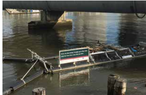
Floating litter trap on the Yarra River in the Docklands precinct. Photo: A Kilborn
