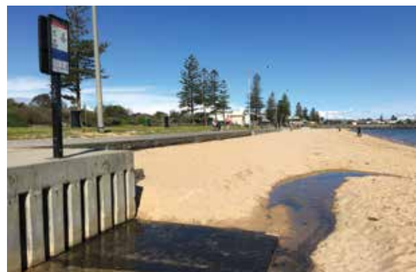
Urban stormwater drain at Elwood Beach. Photo: R Molloy
