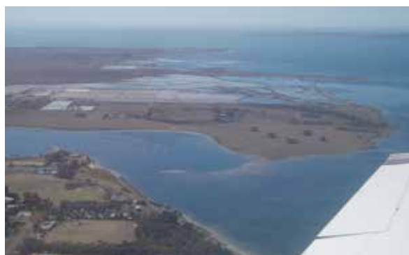
Cheetham saltworks at Avalon, with Limeburners Bay in the foreground. Photo: R Molloy
