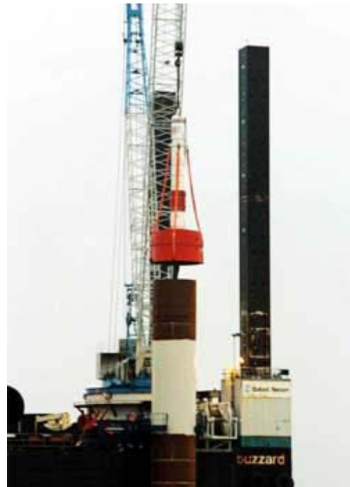
Figure 3. Jack-up rig Buzzard during ramming operation
