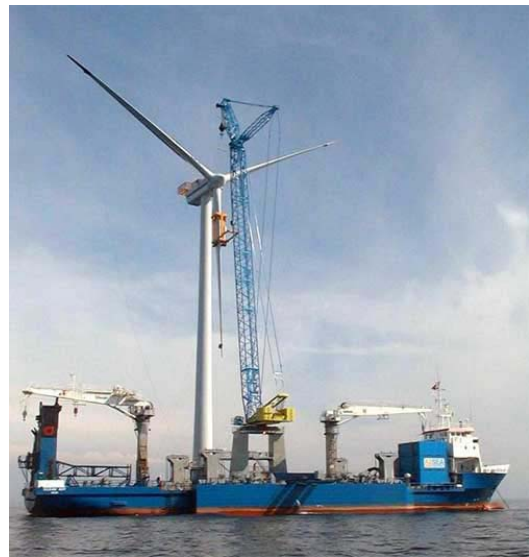
Figur 23 Mounting of wind turbine
