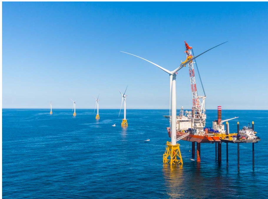
Figure 3.3. Typical example of 6 MW turbines mounted on jacket foundations. Source: Block Island offshore wind farm, US.
