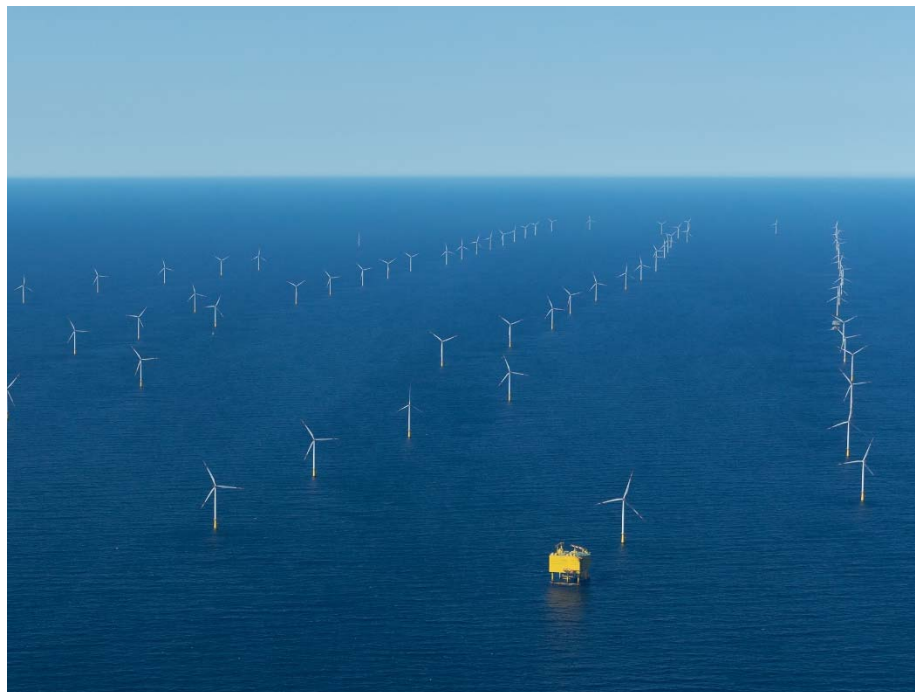
Figure 3.5. Example of operational offshore wind farm (Dan-Tysk, German Bight). Yellow platform in the foreground is the transformer station, which connects cables from all turbines with the main cable to shore. Distance between rows of turbines is roughly 1 km. Source: Vattenfall.
