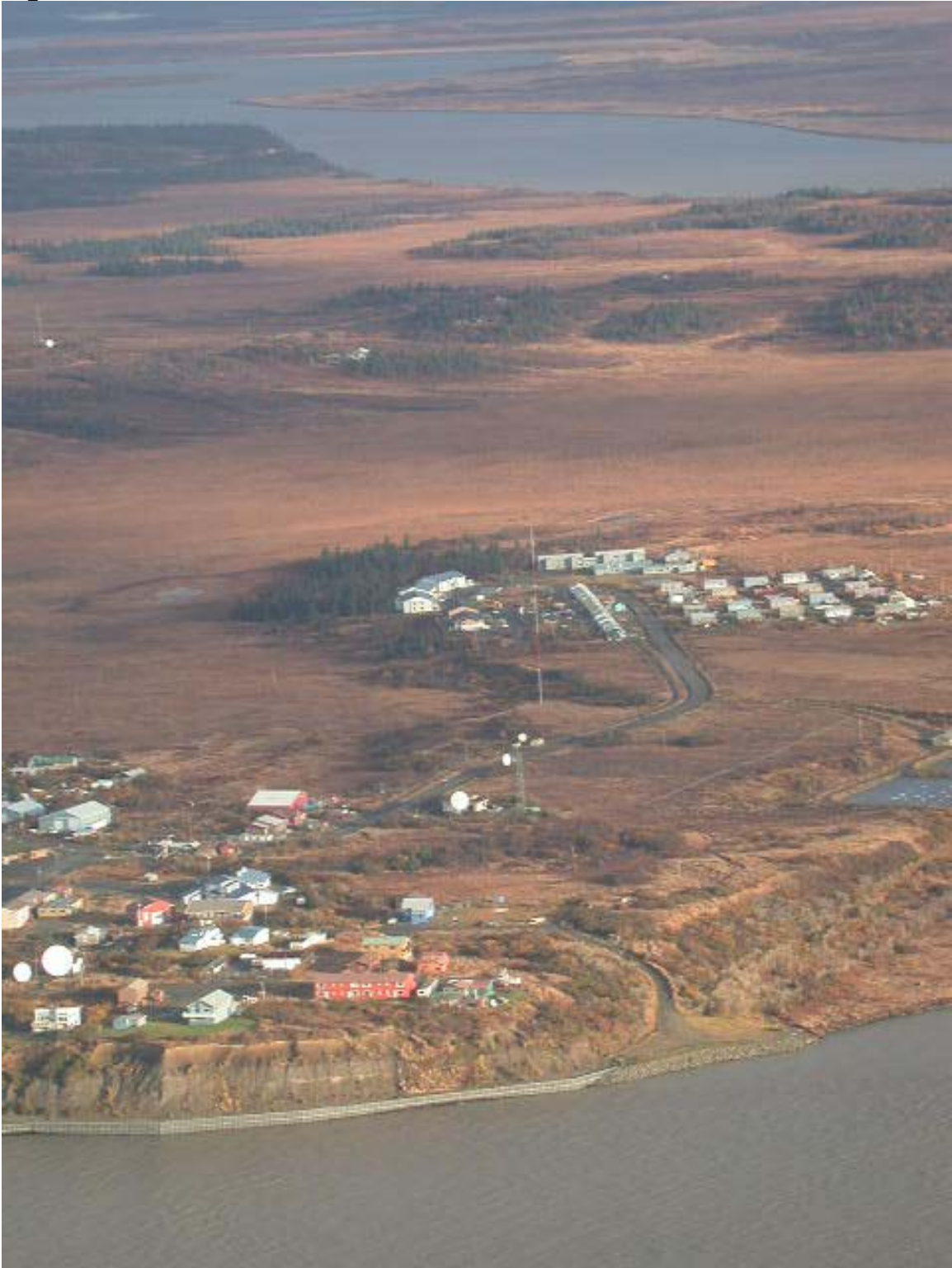
Figure 7 shows an aerial view near the Wood River Road site.
