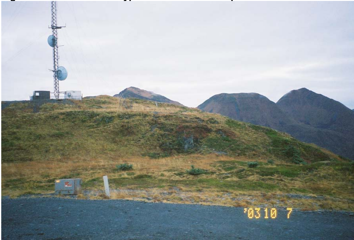
Figure 4 shows a view of typical habitat on the top of Pillar Mountain.
