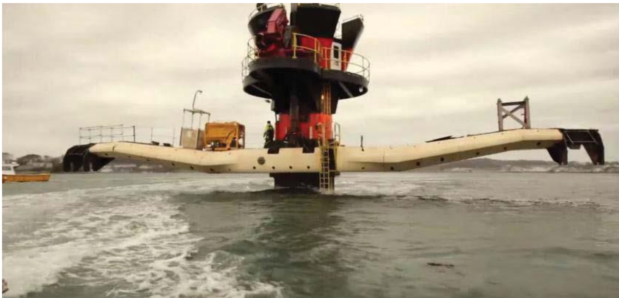
Figure 1.2: SeaGen Device in Strangford Lough with Powertrains Removed (From: SeaGen, 2016)
