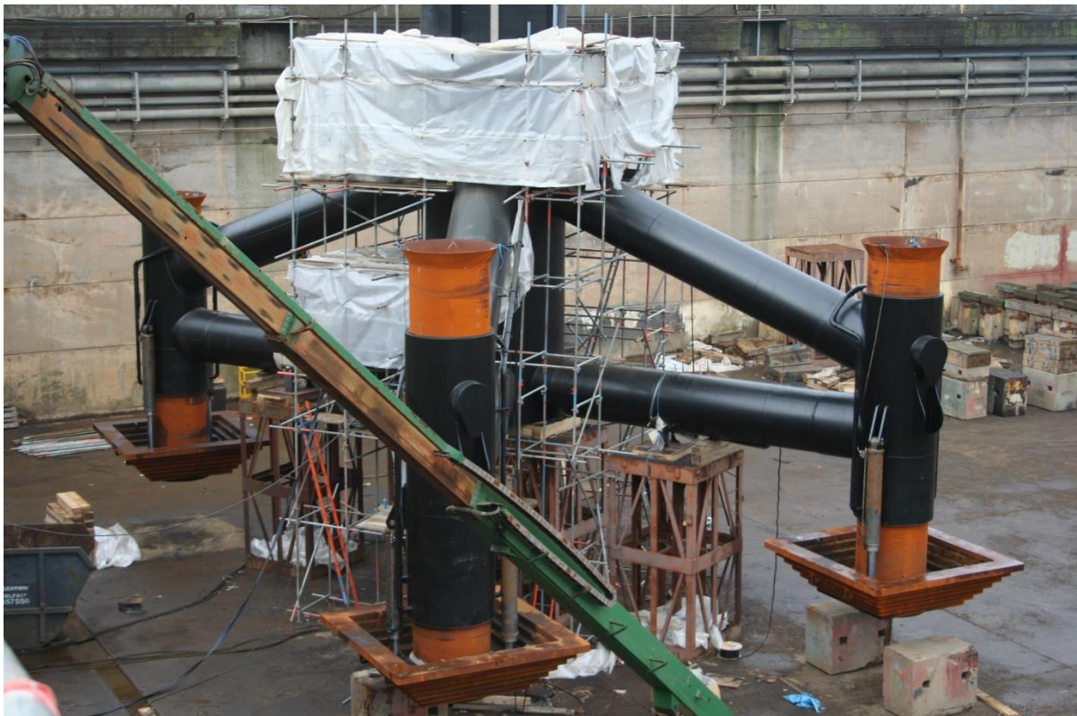
Figure 4.2: Image showing the base of the SeaGen device including the four feet (Image provided by SGL, 2016)
