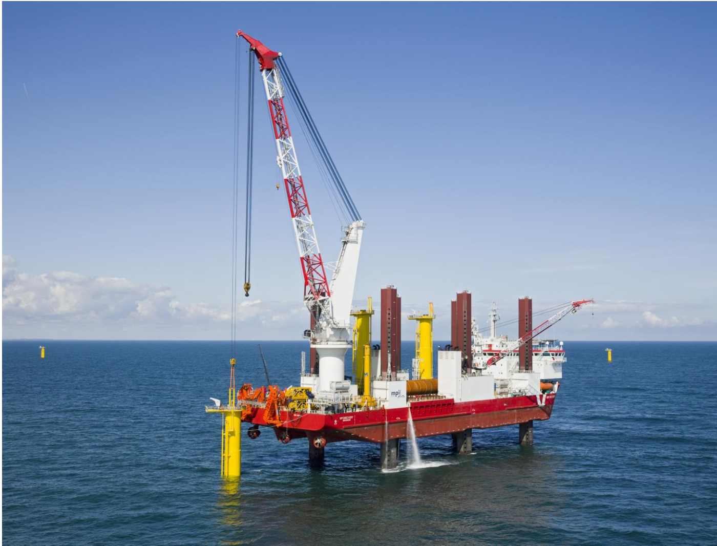
Figure 5: Installation of Transition pieces
