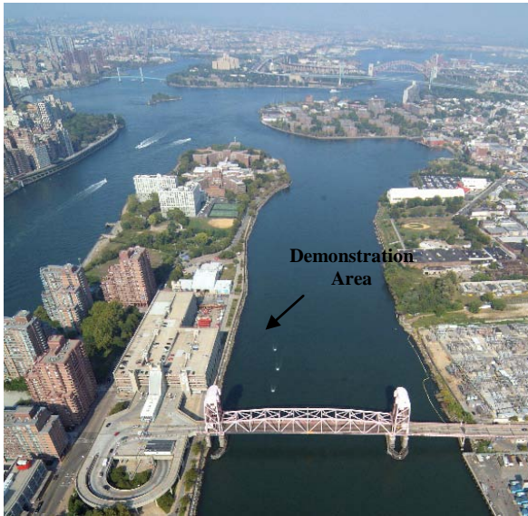
Fig. 3 - RITE Demonstration Site (Aerial View)
