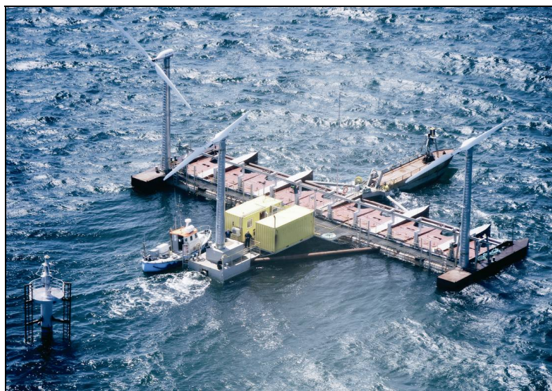
Figure 1-5: Wave Depletion behind Poseidon WEC
