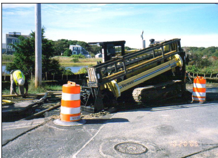
Figure 3-36: Horizontal Directional Drilling in Progress
