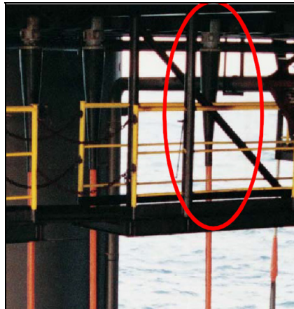
Figure 3-54: Cable Stiffener for Attachment to Off-shore Platform In Situ (Marc Jeroense, ABB AB High Voltage Cables)
