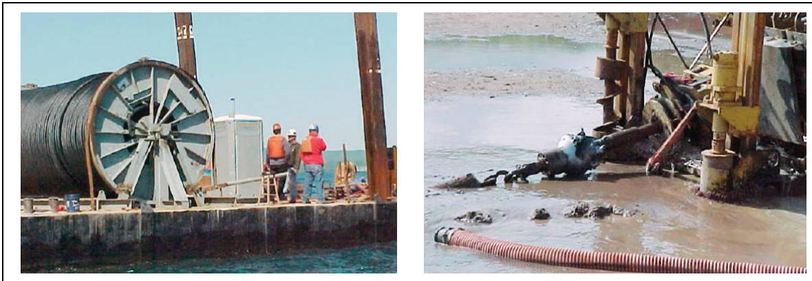
Figure 3-38: Madeline Island Cable Installation ( www.kerite.com )
