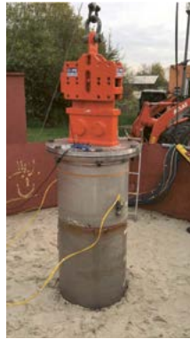
Fig. 2 Vibratory extraction with an Ape Model 3 vibrator of Cape Holland
