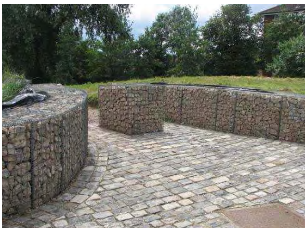
Figure 7 Typical Gabion System
