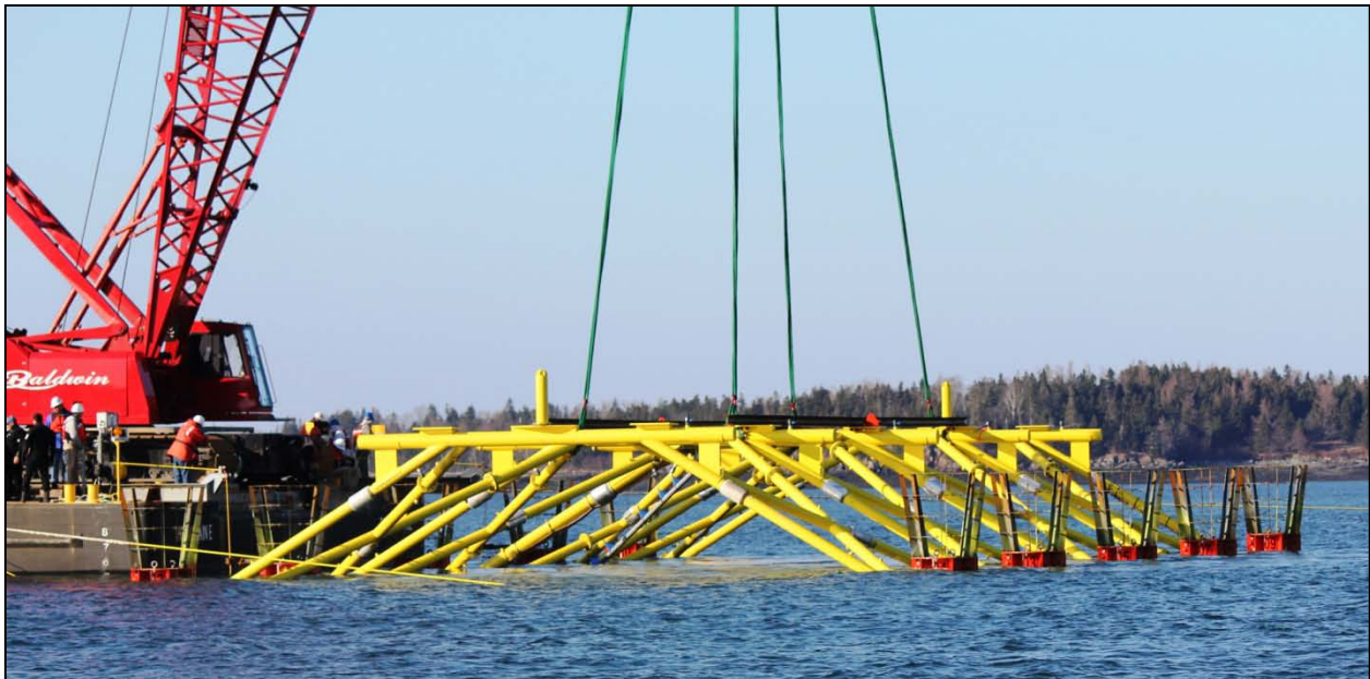
Figure 12. Bottom support frame deployment, March 20, 2012.
