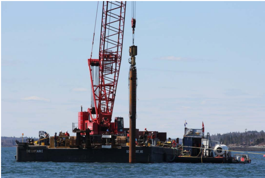
Figure 13. Vibratory hammer operations, April 1, 2012.
