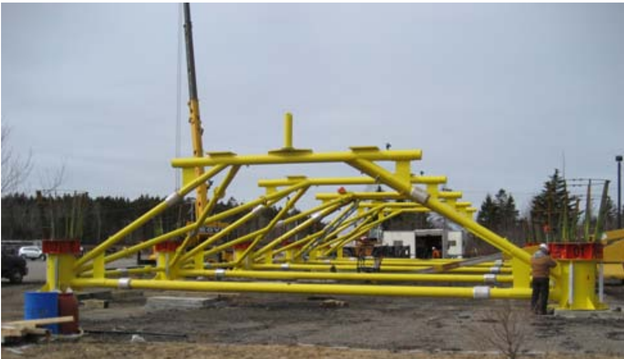
Figure 11. Final assembly of the bottom support frame, March 16, 2012.
