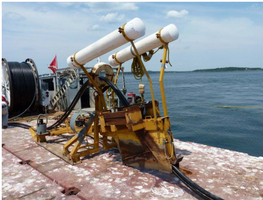
Figure 15. Shear plow used for cable installation (July 13, 2012)
