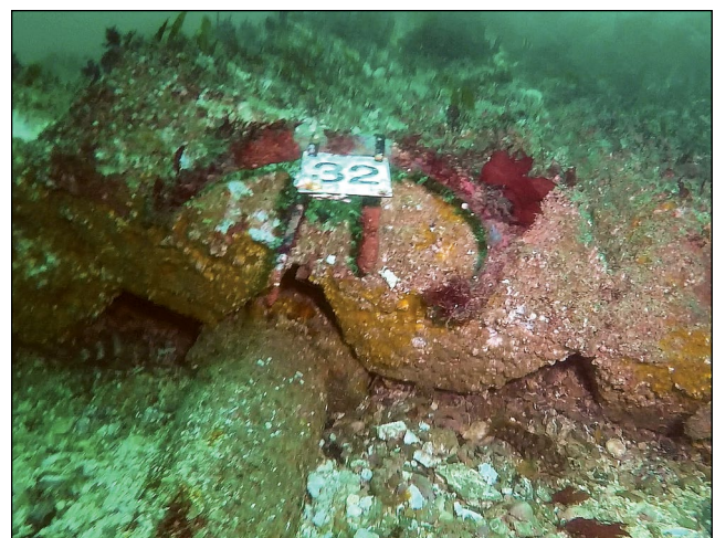
Figure 6.2. Pictures of iron shells and concrete mattresses used to protect an unburied cable at the Paimpol-Bréhat tidal turbine test site in France. The picture on the left was taken one month after the installation of the concrete mattress in 2013 (photo courtesy of Olivier Dugornay, Ifremer), and the picture on the right was taken six years later during a video survey (photo courtesy of Ifremer).
