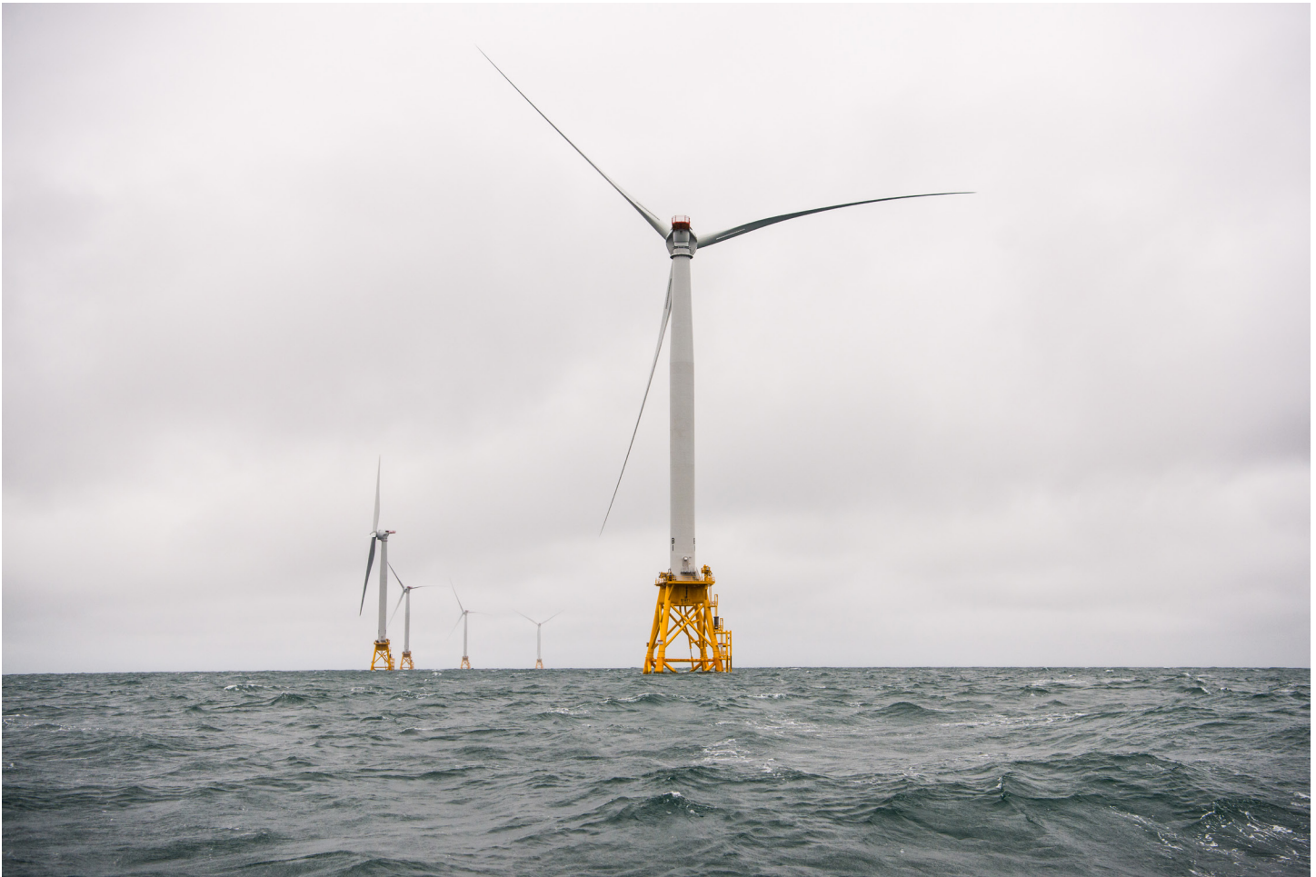
Block Island Wind Farm, Rhode Island (Credit: U.S. Department of Energy)
