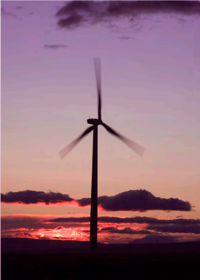
Wind facilities can be shut down temporarily at night during peak migration periods to reduce collisions for bats and birds. Photo © Iberdrola Renewables.
