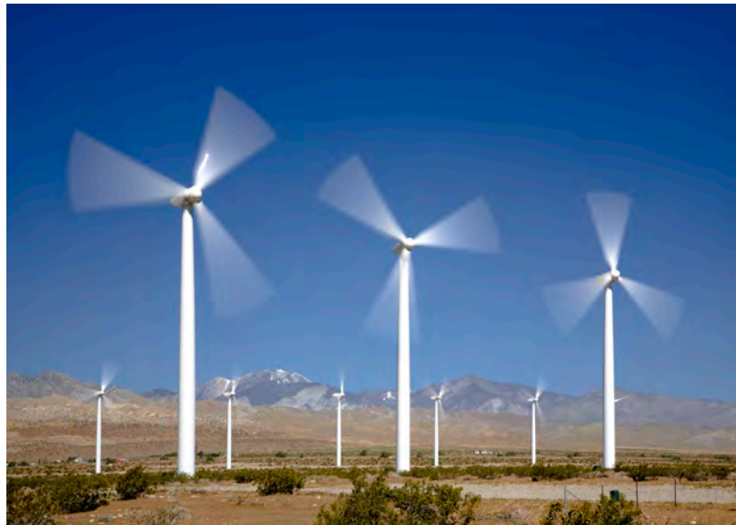
Wind installations affect many bird species. Photo © Iberdrola Renewables.
