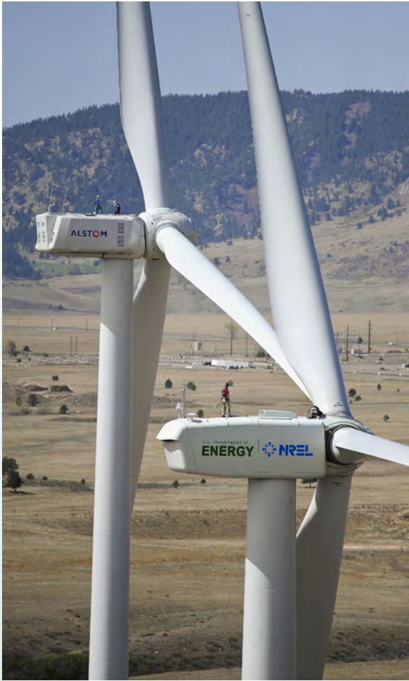
Tubular wind turbine towers are used almost exclusively today and result in less bird mortality than the latticed designs. Photo © DOE/National Renewable Energy Laboratory.
