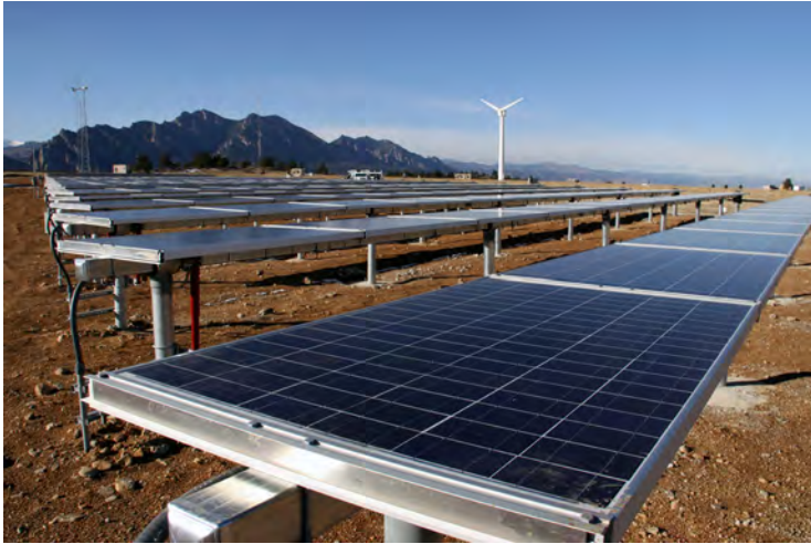
On solar power installations, the site may be cleared of all vegetation to allow access to the installed equipment and to prevent fires. Photo © Joe Verrengia, DOE/National Renewable Energy Laboratory.
