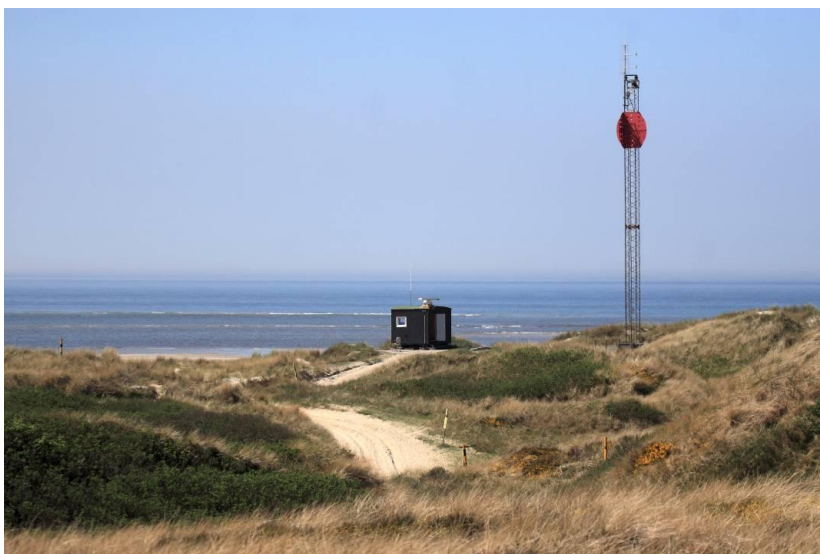
Figure 3-2: The observation platform and mounted radar at Blåvands Huk.
