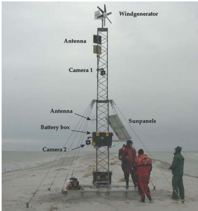
Figure 6.24. Camera tower at Rødsand Seal Sanctuary with antennas, wind generator, solar panels and battery box.
