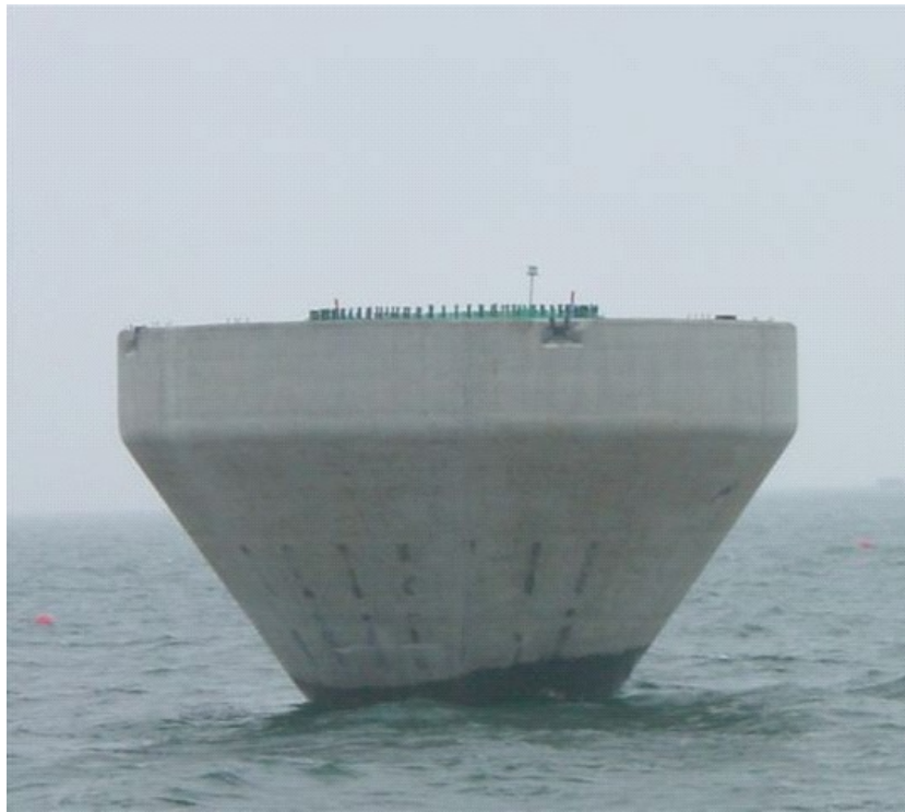
Figure 6.3. Picture of one of the turbine foundations put in position in the wind farm area.
