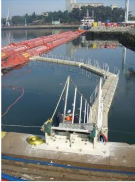
Figure 3.13 Access for light maintenance used in Portugal
