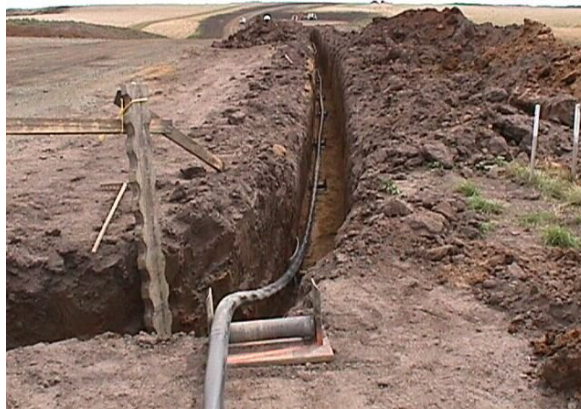
Figure 2.8: Typical 22 kV underground cable installation.
