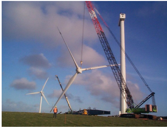
Figure 2.7: Turbine erection - rotor installation.
