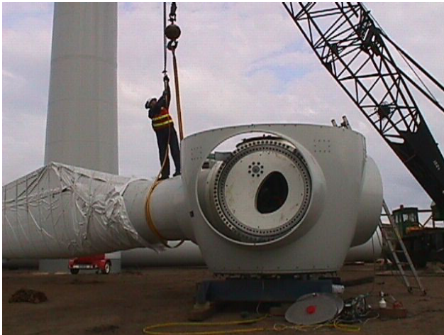
Figure 2.6: Turbine erection - rotor assembly.
