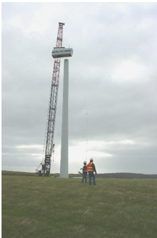
Figure 2.5: Turbine erection - nacelle installation.
