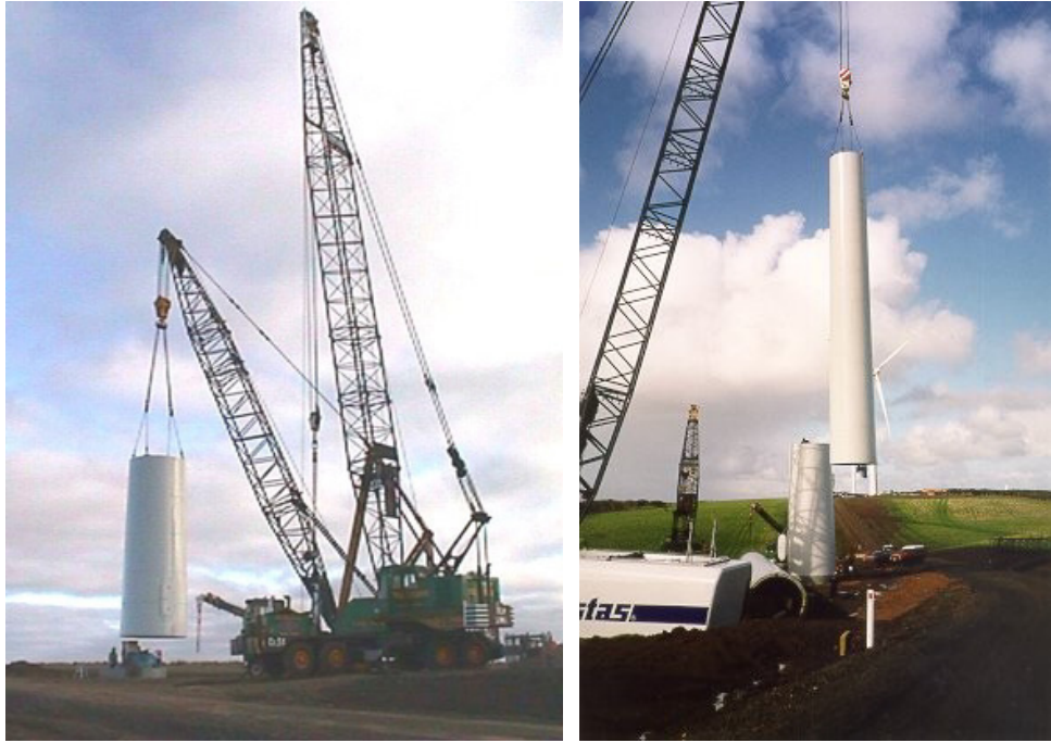
Figure 2.4: Turbine erection - tower installation.
