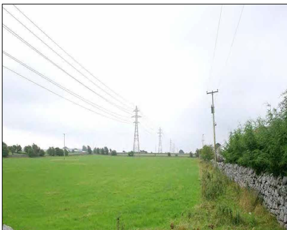
Typical 110 kV double circuit structures
