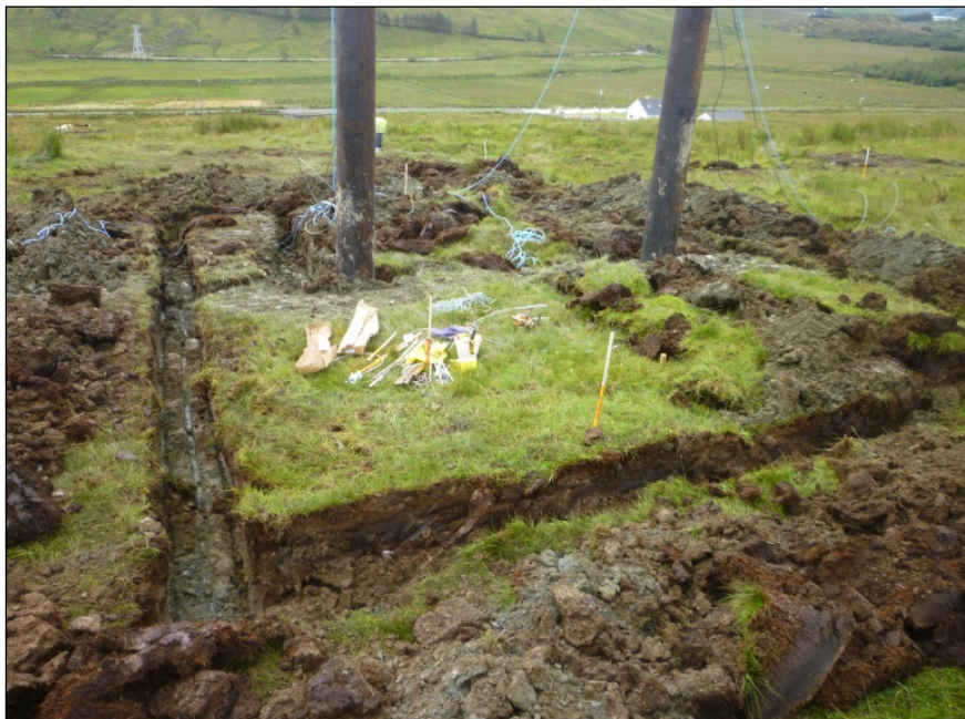
Earth ring on Donegal 110kV Project
