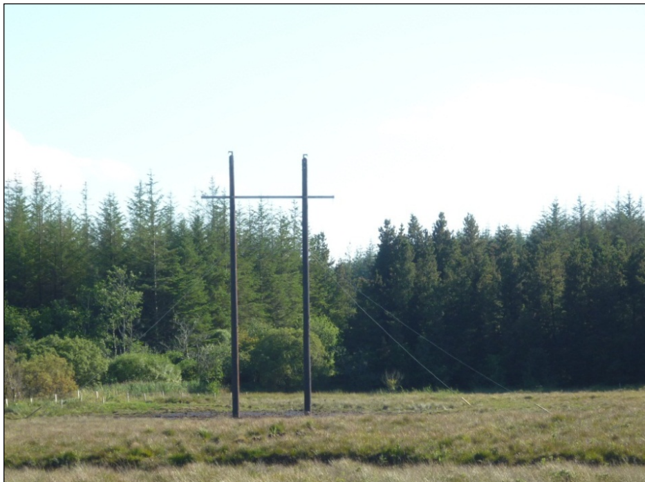
Stay lines in place, Donegal 110 kV Project
