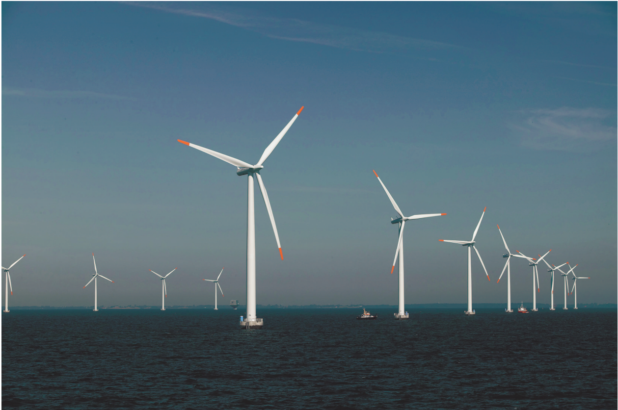
Figure 2 Nysted Offshore Wind Farm. Photo: Energy E2.
