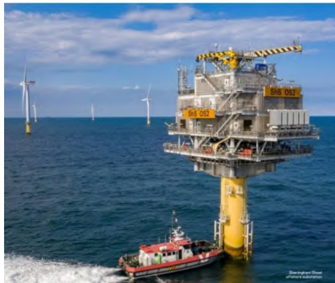
Fig. 1.1.3. Sheringham Shoal offshore transformer substation 7 .
