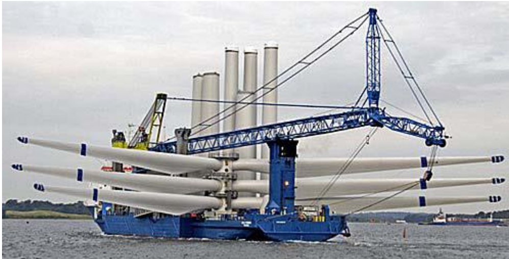
Fig. 1.2.6. The vessel “Sea Power” is shipping wind turbines to the Lillgrund wind farm construction site (photo by Jeppsson et al. 2008).
