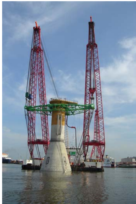
Figure 2. Transport of the first GBF from the port of Ostend to the Thorntonbank (Photo R. Brabant/RBINS).
