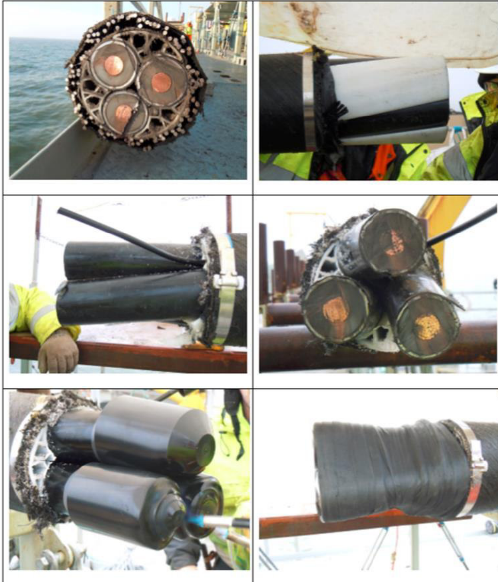
Figure 5.16 - Typical cable cutting and sealing process
