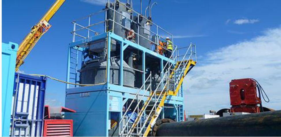
Figure 5.11 - Example of grouting spread set up on a HLV
