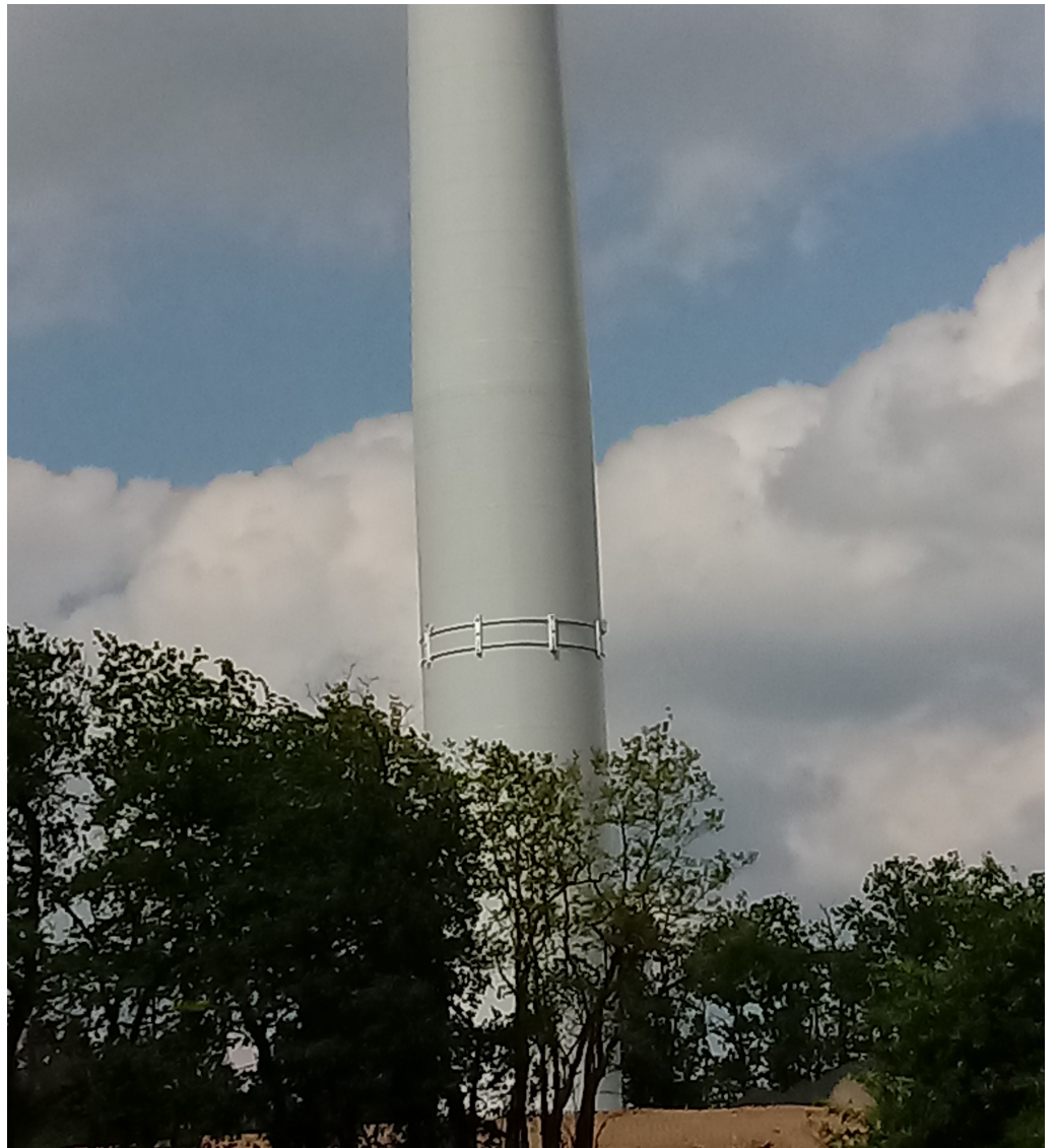
Figure 19. The system prototype mounted on a wind turbine at the test field. The system consists of eight Detection modules fixed on the tower wall and the Decision-making system placed inside the tower.
