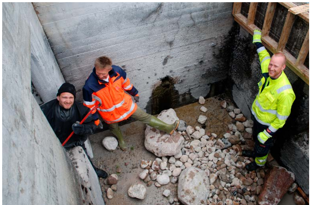
A fishway at Høyegga in the Glomma river has been transformed from a “salmon fishway” to a “vertical-slot fishway” by sawing slots from the top to the bottom of the pools allowing the fish to swim through the holes instead of having to jump. Photo: Jon Museth
