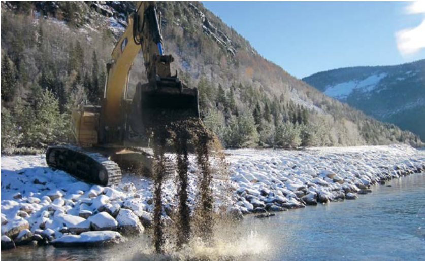
Once a diagnosis has been established practical measures may be undertaken in accordance with detailed descriptions in the handbook. Here, a new spawning area is under construction. Photo: Ulrich Pulg.
