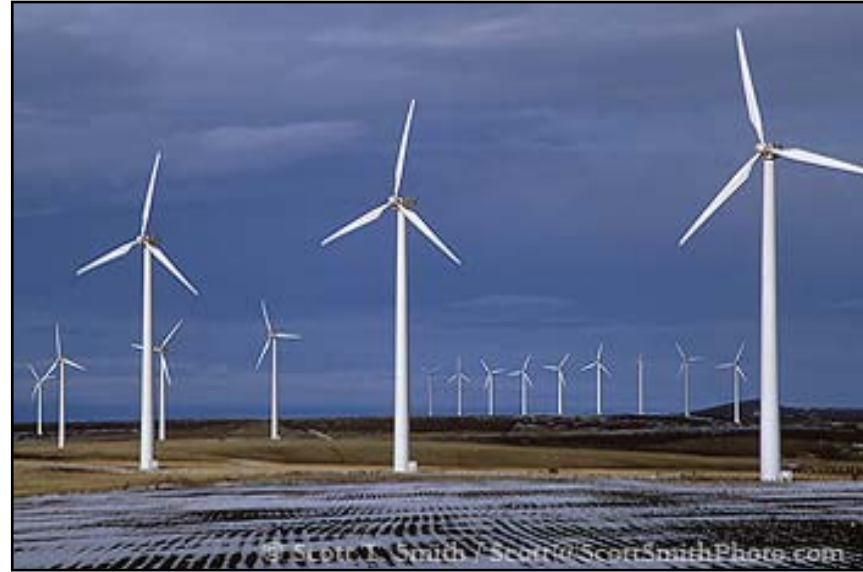
Wind power facility in the dry-land crop fields in eastern Oregon, a compatible use that reduces environmental conflicts. Scott Smith photo.
