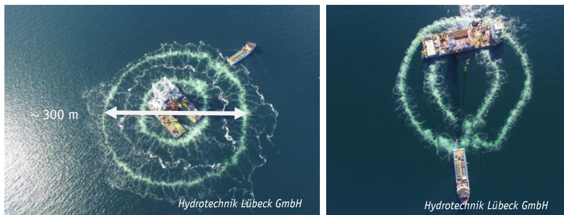
Figure 29: Double Big Bubble Curtain: left: circular deployment due to the very low current; right: elliptic deployment due to the current (larger diameter in current direction). (Source: Hydrotechnik Lübeck GmbH)
