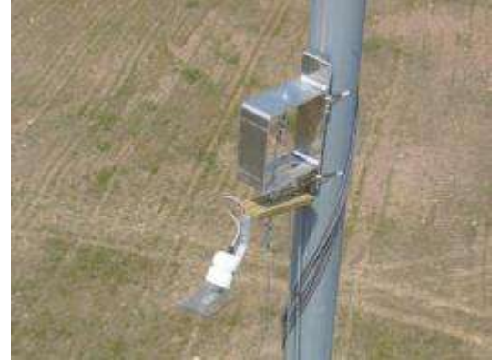
A mounted pulley system and bat hat at 22 m high.
