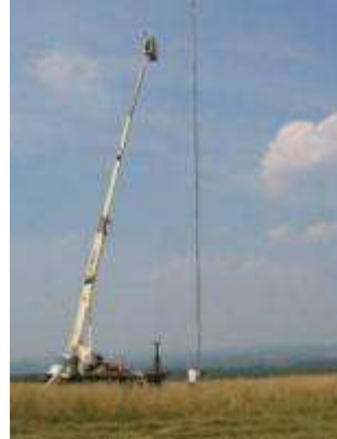
Boom truck used to mount pulley system
