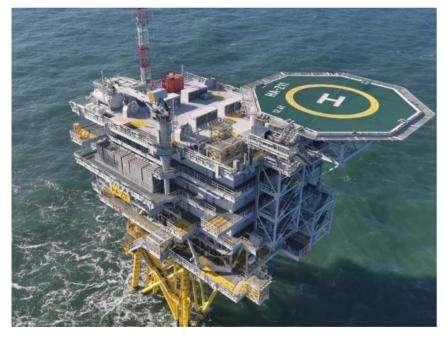
Figure 30 One of the fixed offshore substations used at the Hornsea One project. *Image courtesy of Ørsted. All rights reserved.*
