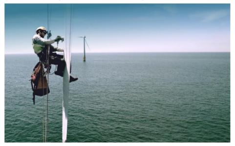
Figure 43 Blade inspection and minor repair being carried out by a ropeaccess technician. *Image courtesy of Altitec. All rights reserved.*
