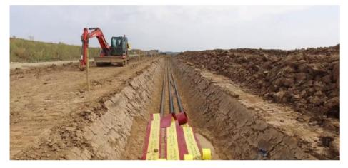
Figure 36 Onshore export cable trenching process. Image courtesy of Ørsted. All rights reserved.
