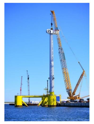
Figure 40 A landside crawler crane lifting a nacelle onto a floating substructure. *Image courtesy of Port Pictures / Danny Cornelissen. All rights reserved.*
