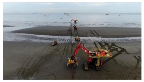
Figure 34 Offshore export cable transitioned to shore. *Image courtesy of Jan de Nul. All rights reserved.*
