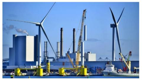
Figure 39 Floating offshore wind turbine final assembly taking place at port. *Photo of the Kincardine Offshore Wind Farm project courtesy of Principle Power.*
