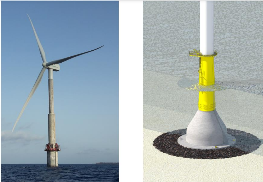
Gravity-Base Structures (GBS)
