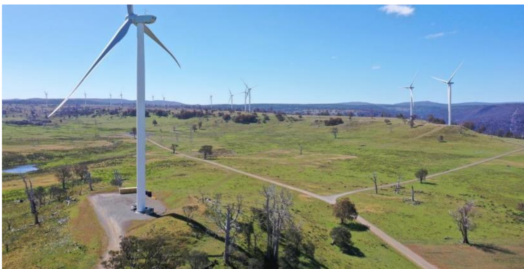
Plate 4: Eastern part of CHWF with turbines on ridgelines west of Ouse River Valley.
