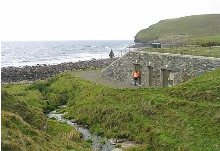
Figure 6: EMEC substation external view.
