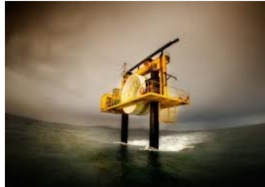
Figure 8: Open Centre Turbine deployed at EMEC
