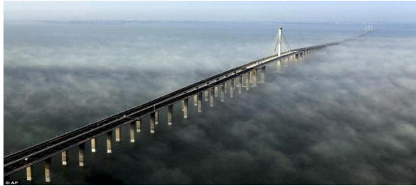
Jiaozhou Bay Bridge ( 26.4 miles long) Dailymail.co.uk
